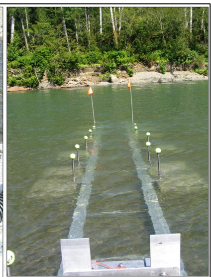
Aluminum track installed in river
